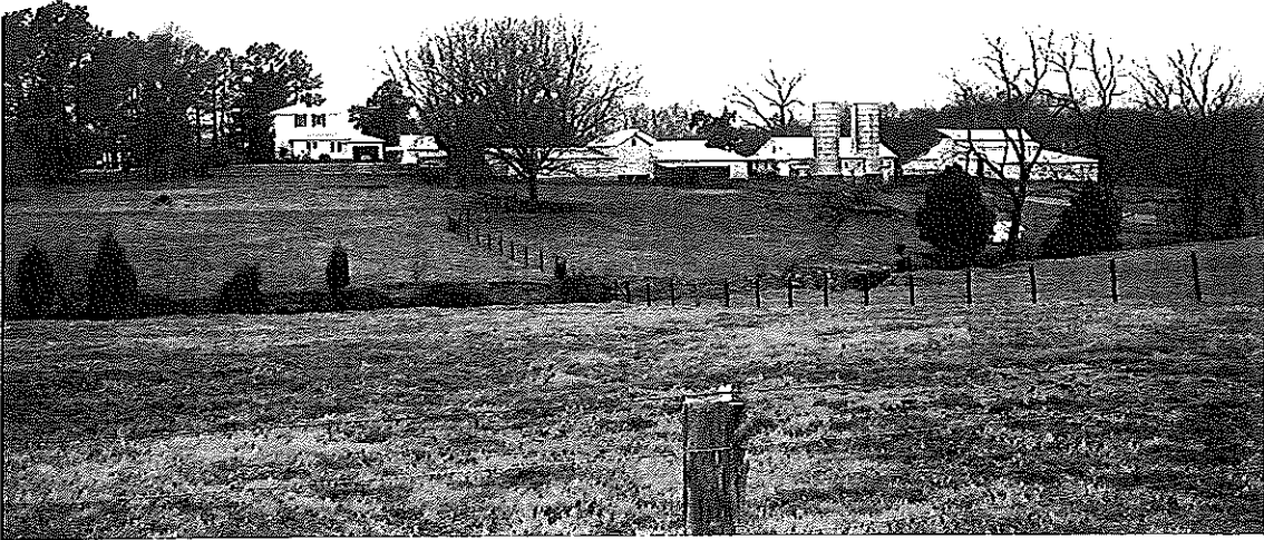
28. Paisley-Cates House. View from the east (Paisley-Cates House is at extreme left; dry creek bed in foreground is part of the proposed National Register boundary).
