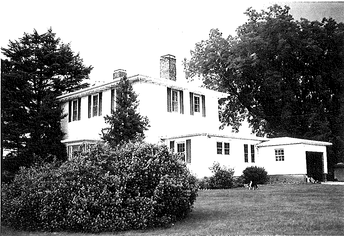
28. Paisley-Cates House. Three-quarter view from southeast.
